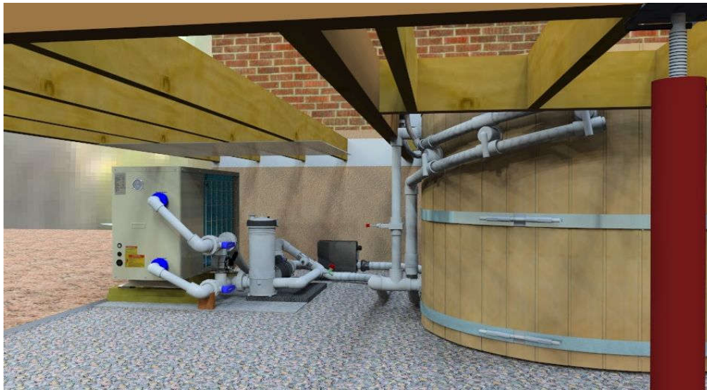
Figure 32 - Typical Stand-alone installation with Heat Pump
